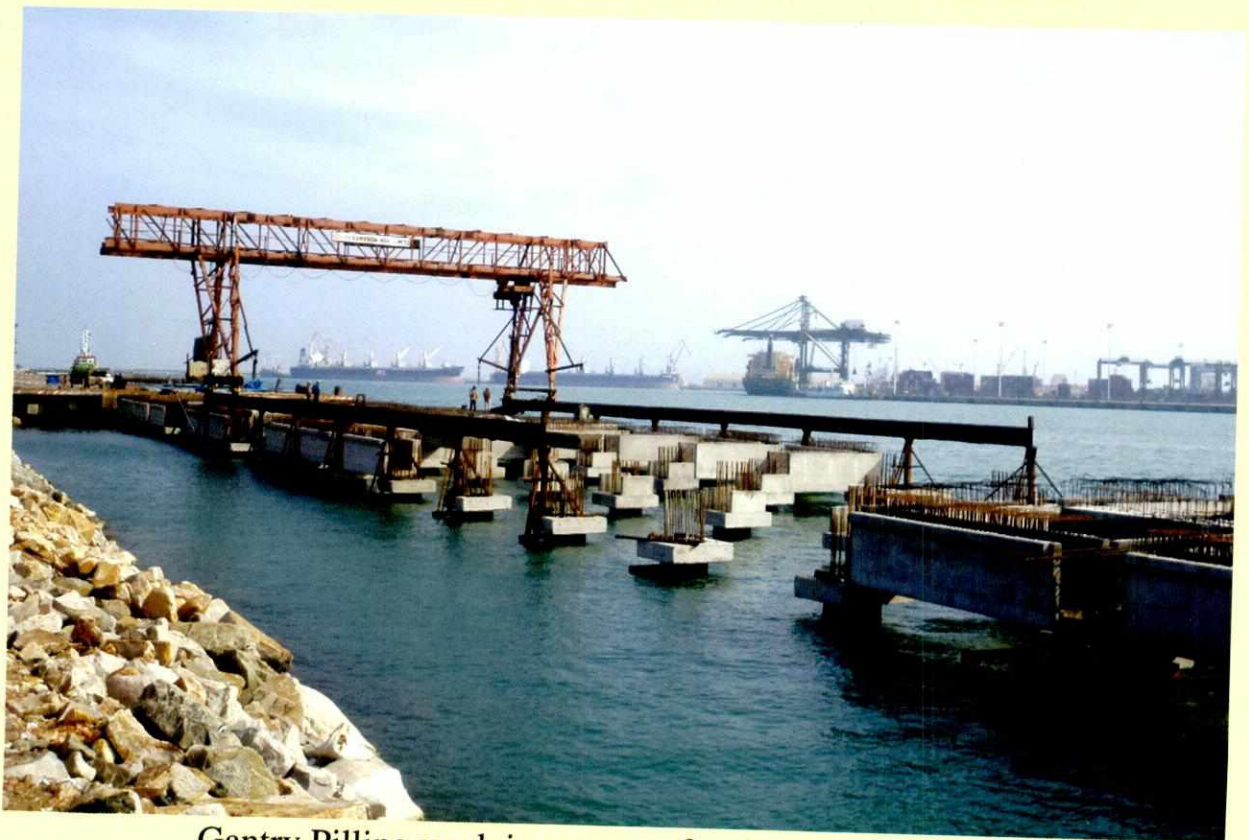
Gantry Pilling work in progress for the Construction of North Cargo Berth II (NCB II) being Developed under PPP mode to create additional capacity of 7.20 MTPA
