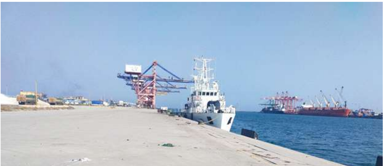
Construction of North Cargo Berth-III with quay length of 306 metres was completed at a cost of ₹ 35.24 crore
