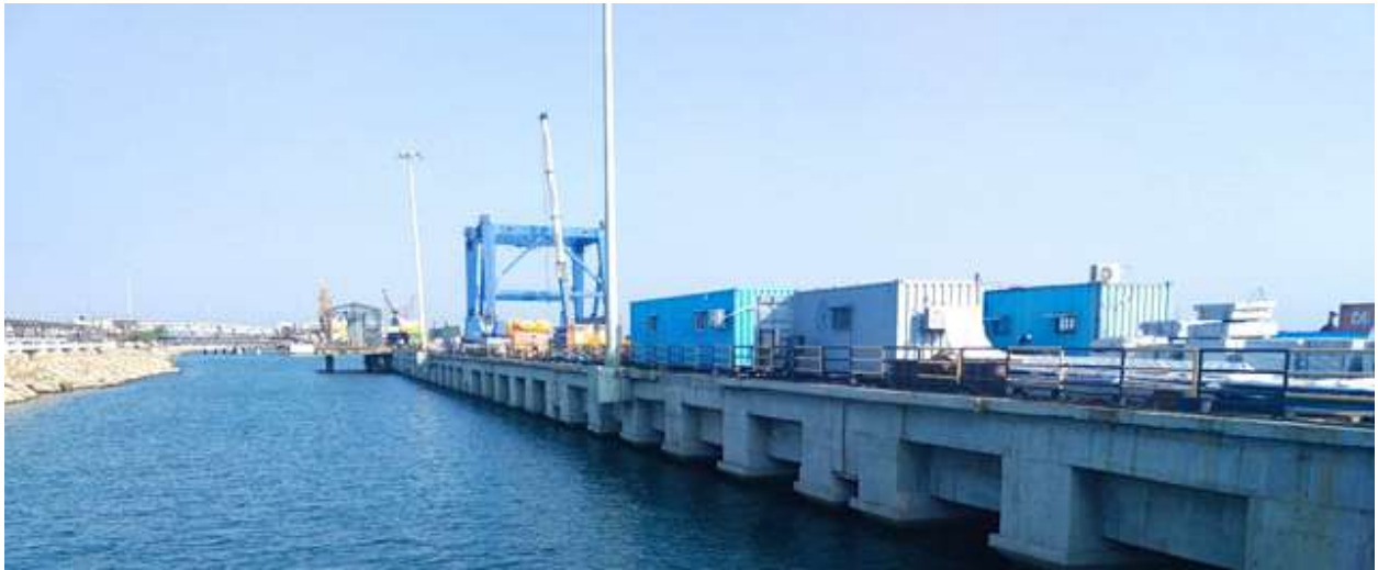
Upgraded Coal Jetty-I to handle fully loaded panamax vessels having draft upto 13 metres
