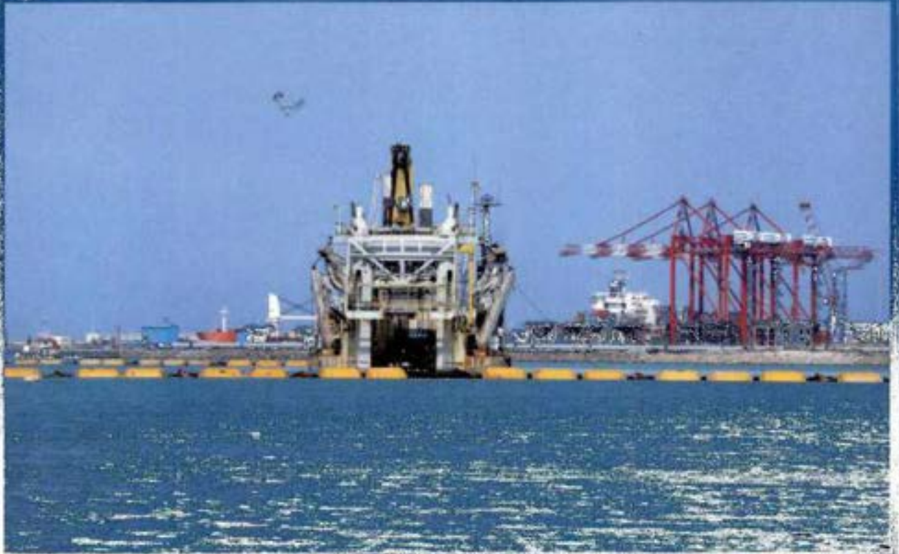
Dredging in front of North Cargo Berth - II
