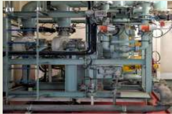
BWTS installed on SCI VLCC DESH VIRAT
