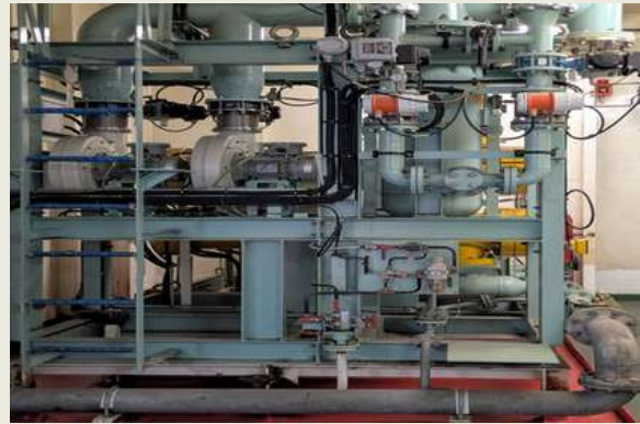
BWTS installed on SCI VLCC DESH VIRAT
